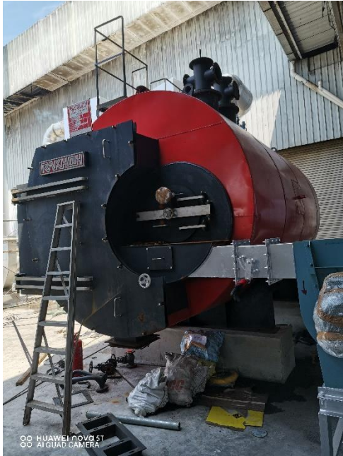
BIOMASS BOILER INSTALLATION
